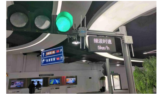
ZTE RSU Demonstrated in Internet of Vehicles Pilot Zone in Wuxi, Zhejiang Province
