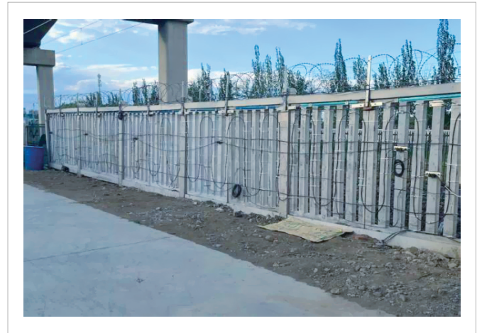
▲ Figure 3. Fiber laying scenario
